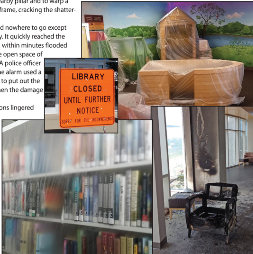
Clockwise from top: Smart Play Area pieces are wrapped after cleaning. The immediate fire area. Restoration workers wrapped shelves and equipment in plastic as they worked from scaffolding to replace ceiling tiles. Signage informed visitors the library was closed.
